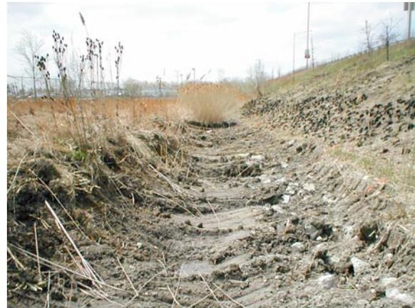
The gasoline plume in the ditch area had migrated approximately ½ mile. Vacuum trucks were positioned in key areas along the ditch line and wetlands to remove the gasoline that had accumulated in those areas. All gasoline and water that was pumped from the ditch and wetlands was transferred to bulk storage tank trailers for off-site reclamation.
